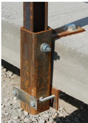
Figure 2. MGS Bridge Rail Installation
